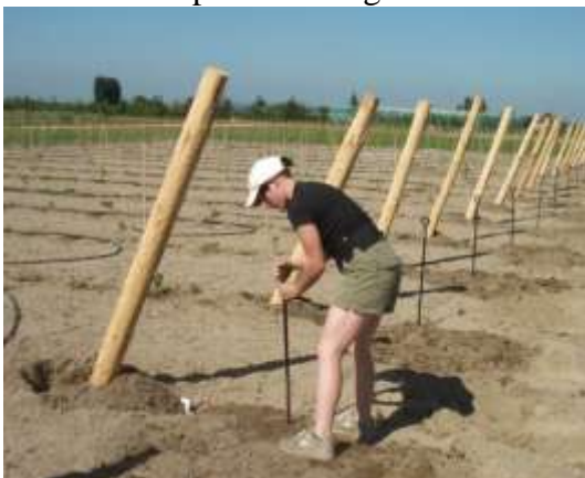
Figure 7. Setting post anchors
