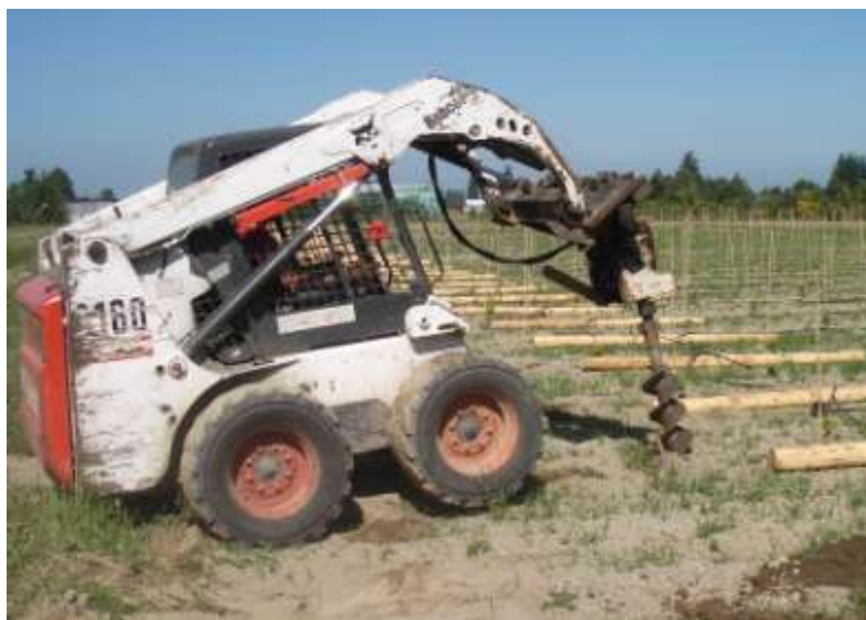
Figure 1. Drilling postholes for end posts
