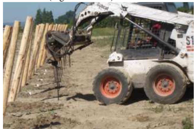
Figure 8. Drilling in post anchors
